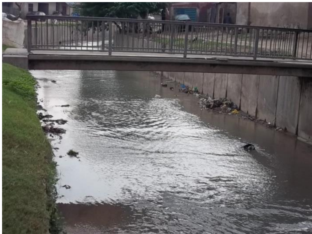
Plate 4. The drainage channel along Kateren Gwari area of Minna.
